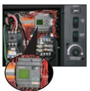
The 1800 Series can be customized to your needs with the standard Smart Relay Control system, which provides complete control over run time, auto start/stop and time delay shut down functionality.
